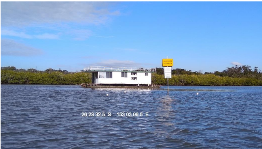
5. HOUSEBOAT ANCHORED AND AGROUND, SCHEDULED FOR DEMOLITION
